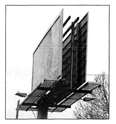
Figure 30.27.095(2) V-type Sign Structure
