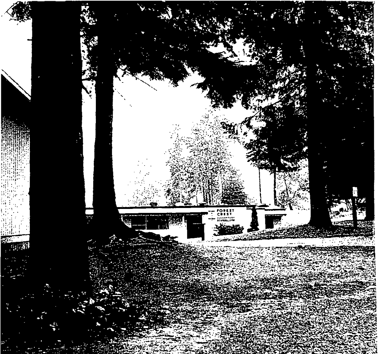
Former Forest Crest Elementary 1956
